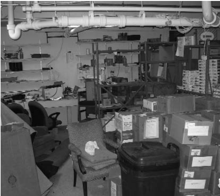
Spring 2006: basement storage area before the start of renovations.
